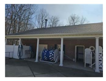
Siding and Trim. The pool house contains vinyl siding and vinyl ceiling. The vinyl appears to be in good condition.
